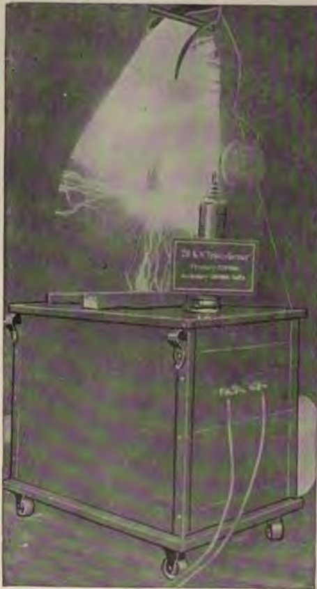
Transformer Discharging Between Sheets of Tinfoil Around a Glass Plate.
